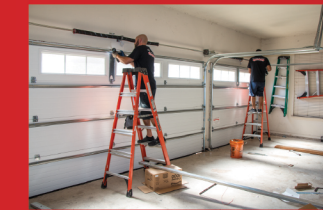
Professional Service & Installation
